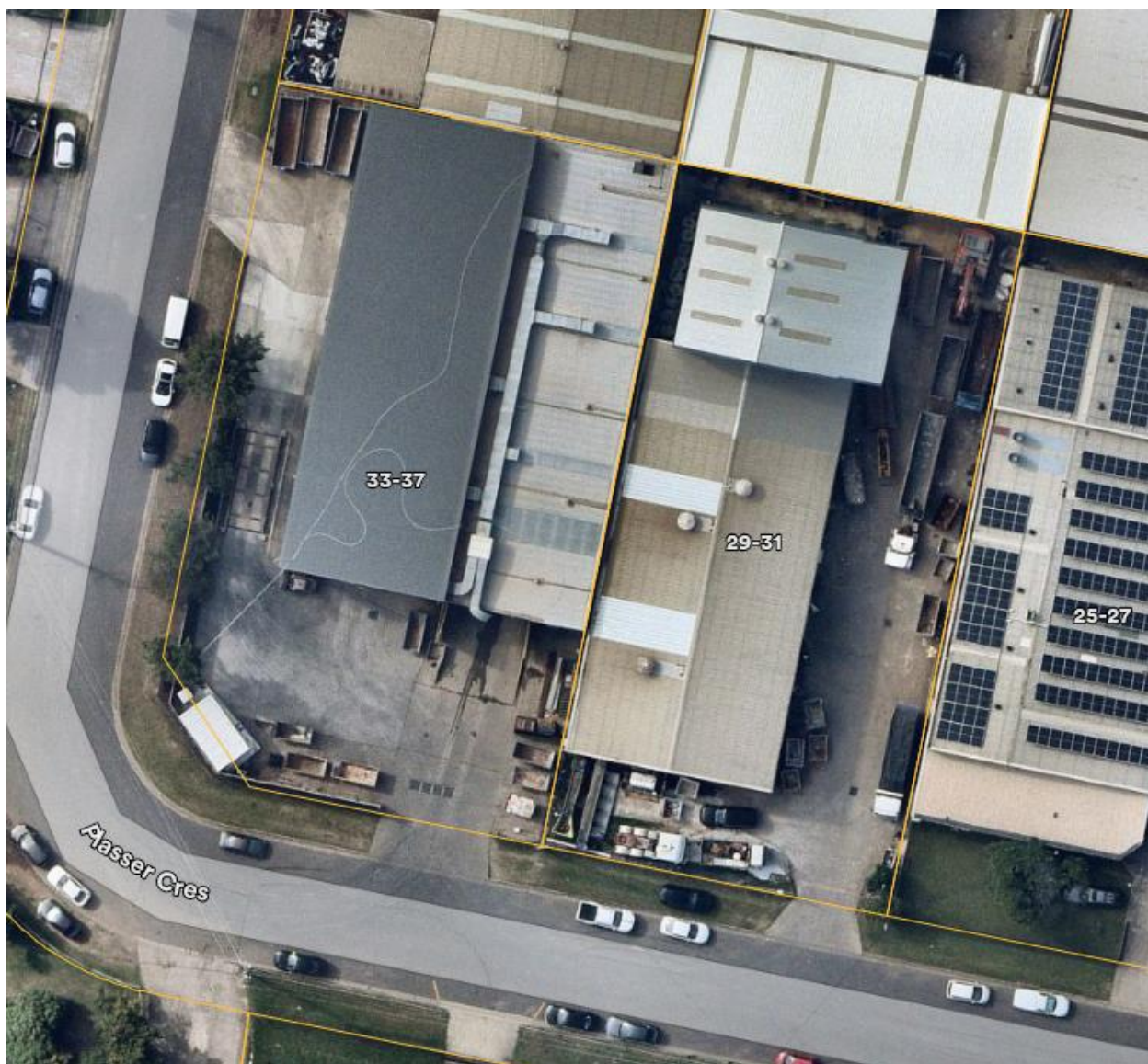
Figure 2 Close up view of the site
